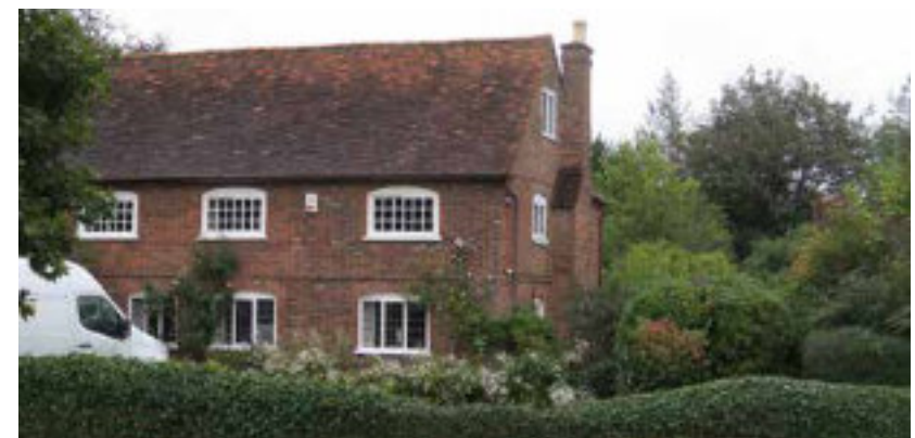
Green End Farmhouse - red brick façade with upper floor horizontal sliding sash windows and ground floor multi-paned casement windows with cambered heads.
