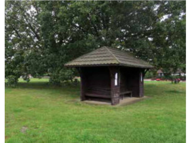
Figure 80: Timbershelter on the Green.
