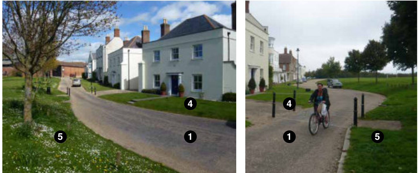
Figure 42: Examples of edge lanes in Dorchester, with low-speed roads shared between motor vehicles and cyclists, and opportunities for on-street parking (note: some localities may prefer clearly defined footways and parking bays).
