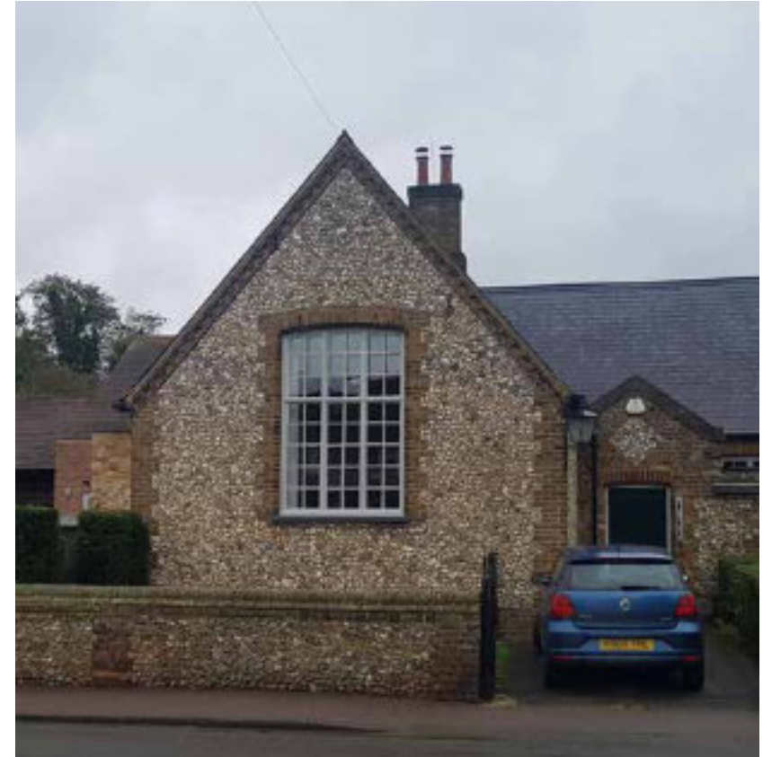
Quoins and window trims in yellow stock brick with knapped flint infilling. Detailed brickwork highlighting eaves and house entrance. Boundary wall with matching materials.
