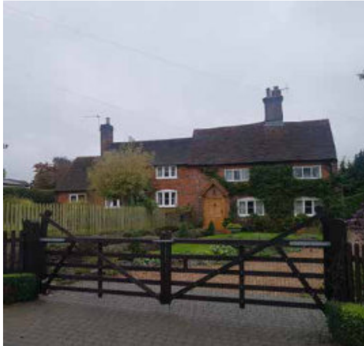
Figure 11: Red brick building with clay plaintile roof.
