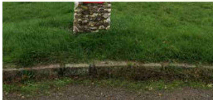
Figure 78: Granite kerbs along the Green.
