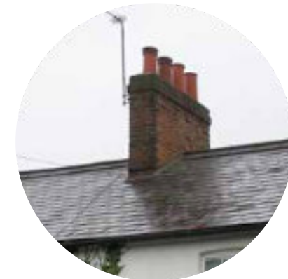
Red brick chimney
