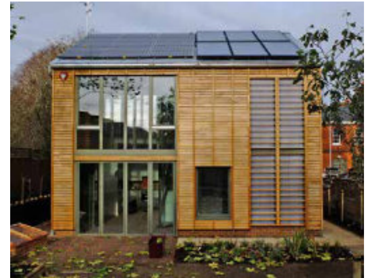
Figure 83: Example of eco design led architecture.
