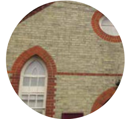
Red brick trim and yellow brick infilling
