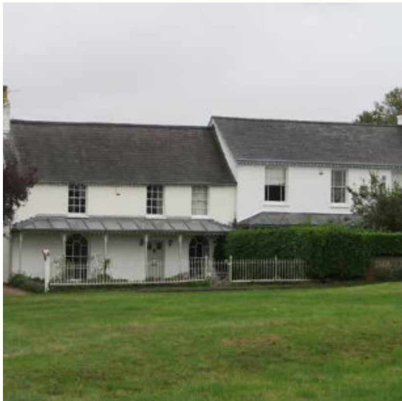
Sarratt House (left) and the White Cottage (right), two listed houses with prominent verandahs (front garden cast-iron railings of Sarratt House also listed).
