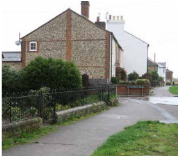
Figure 17: Houses along the Green showing a variety of building recesses and front yard depths.
