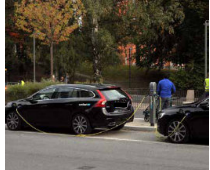
Figure 60: Inset parking with electric vehicle charging points.
