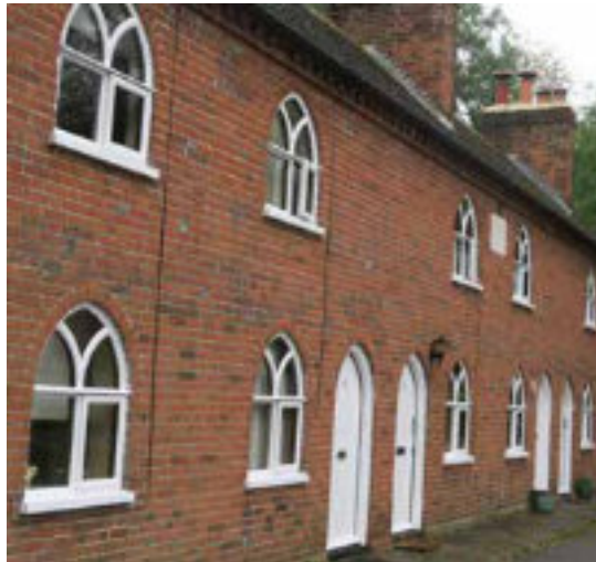
Consistency of arched window and door shapes across the main elevation.
