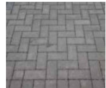
Dark grey concrete block paving
