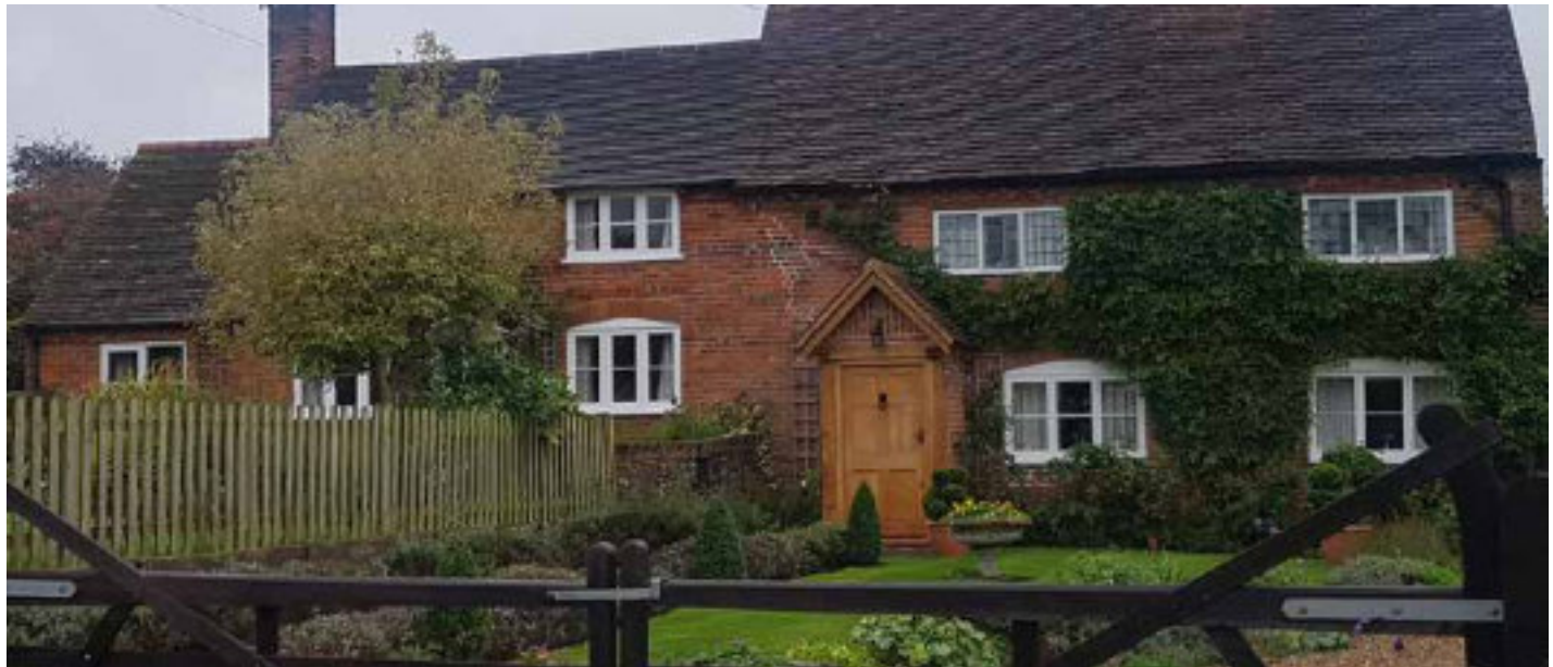
Figure 70: Traditional house with upper floor horizontal sliding multi-pane sash windows and ground floor casement windows with cambered heads.
