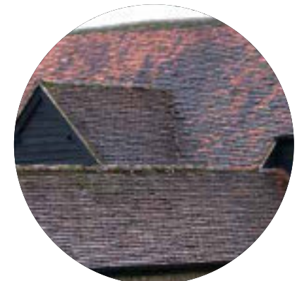
Clay pantiler roof
