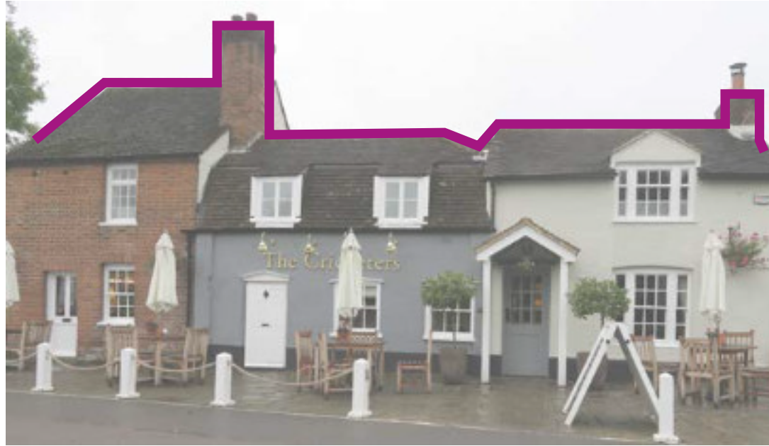
Figure 27: A group of buildings exhibiting a variety of roof heights types. The purple line highlights roofline variations.
