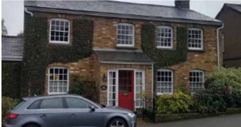
Yellowstock brick house with symmetrical elevation emphasised by an even distribution of sash windows and consistent treatment of window details.
