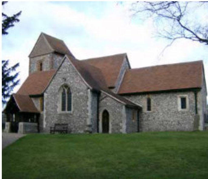
Figure 8: Church of the Holy Cross (late 12th century) - knapped flint infill, ashlar and red brick quoins, and clay plain tile roof.
